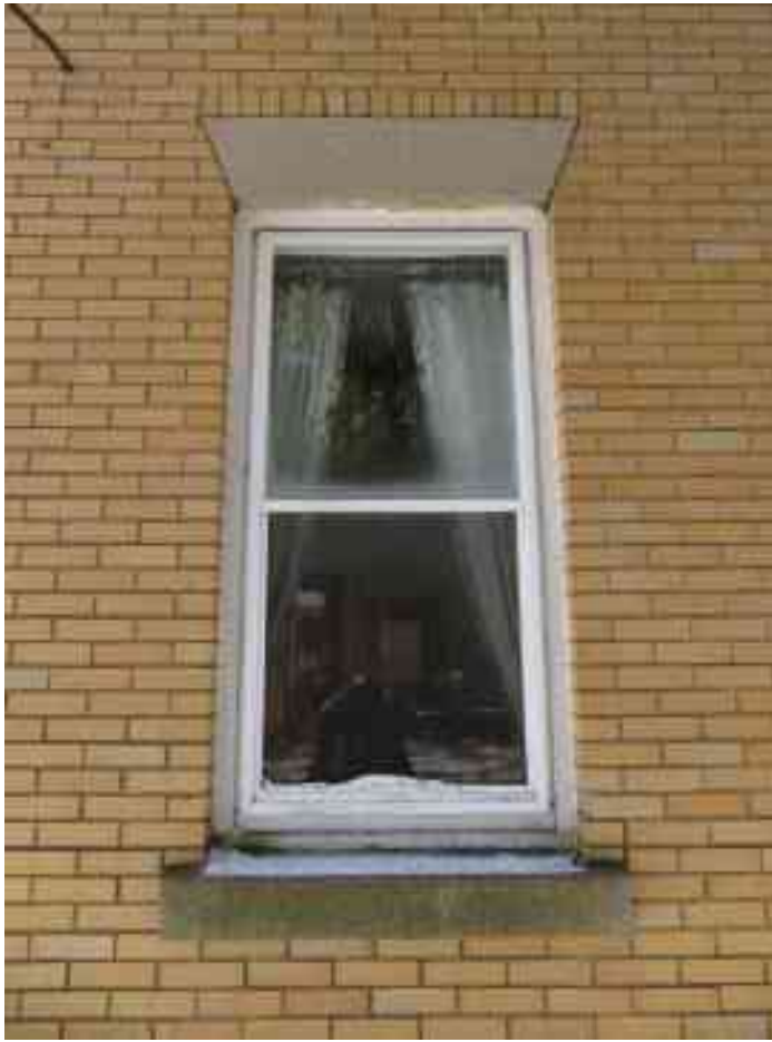
Photo 10.5: (left) Detail at exterior of typical window with an exterior aluminum storm window unit.
