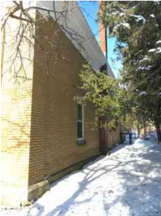
Photo 05: Looking southwesterly at front entry. Note that concrete walk has sunken to create shallow step at access to front doors.
