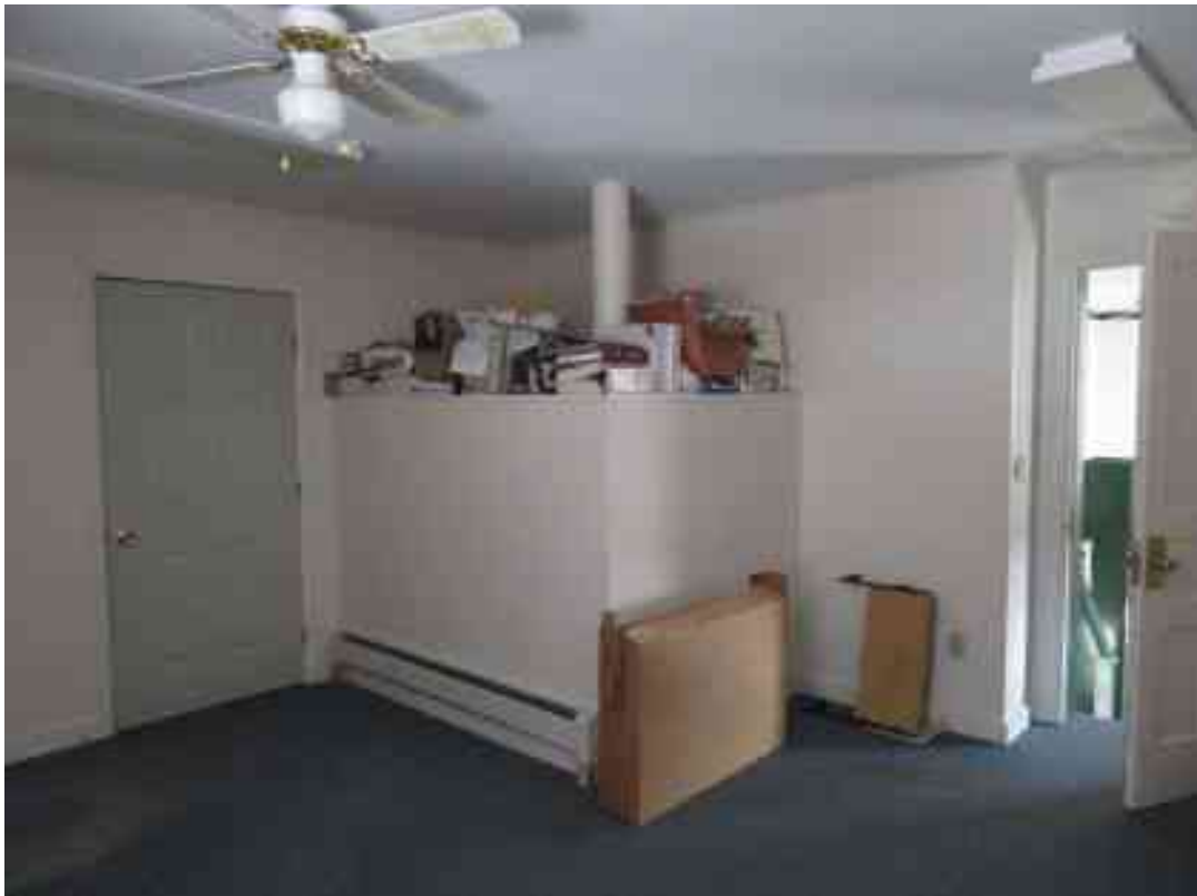
Photo 21: (below) Looking northeasterly in Southwest Room, stage level, towards Toilet Room enclosure.
