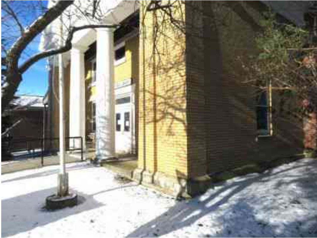
Photo 05: Looking southwesterly at front entry. Note that concrete walk has sunken to create shallow step at access to front doors.
