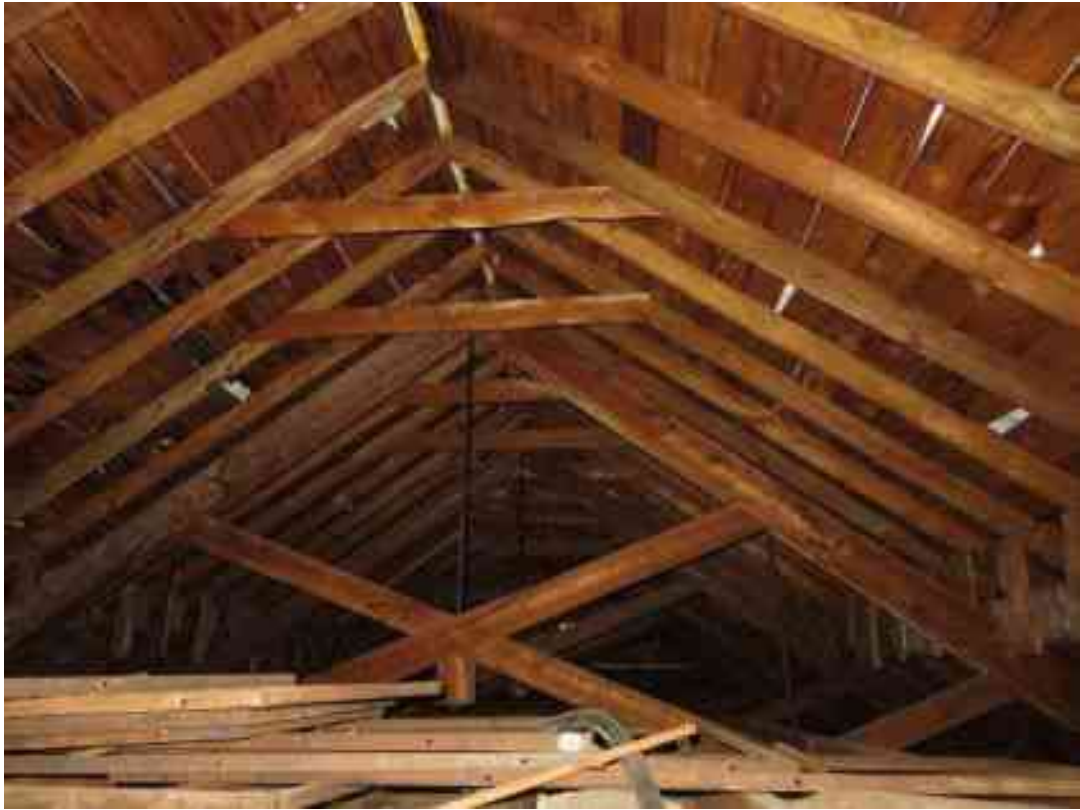
Photo 28: View of primary roof framing in attic.
