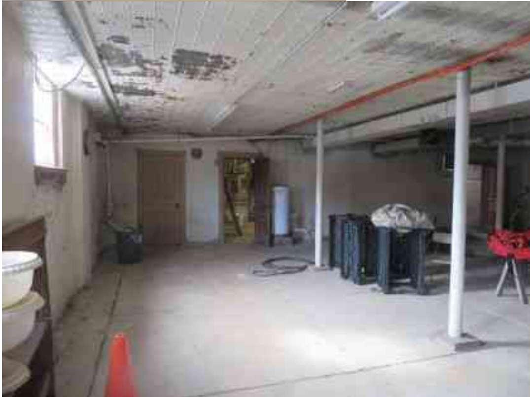
Photo 36: (below) Looking west in Center Basement. Note water heater and exposed mechanicals.
