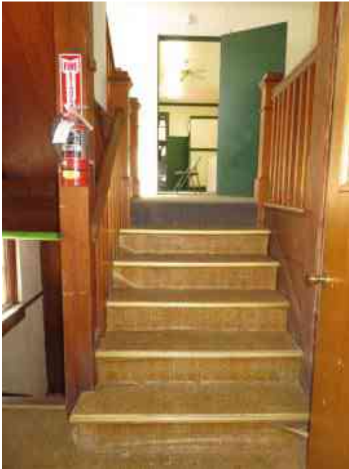
Photo 16: (left) Looking westerly up historic stair to main level.
