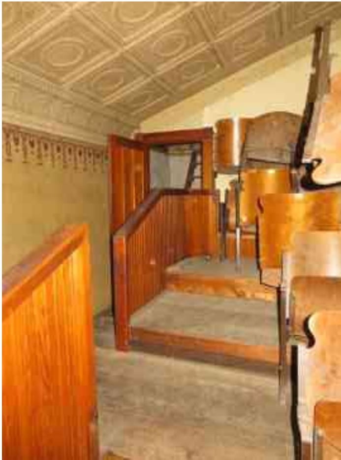
Photo 24.2: (left) Looking northeast in northeast corner of balcony.
