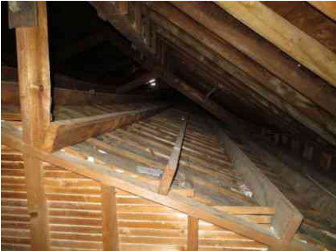
Photo 28.1: Top of theater ceiling framing, attic space, and roof framing above.
