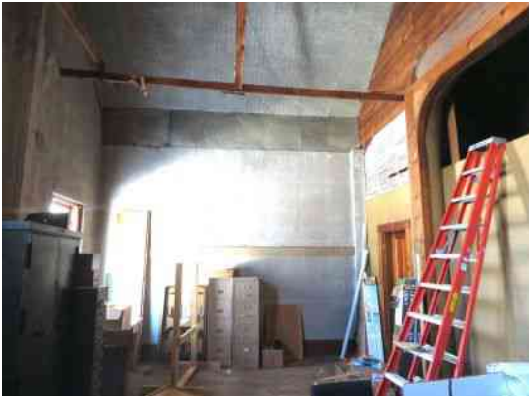
Photo 23: (below) Looking north in Storage Room, stage level. Note ladder access to space above level added within original theater.
