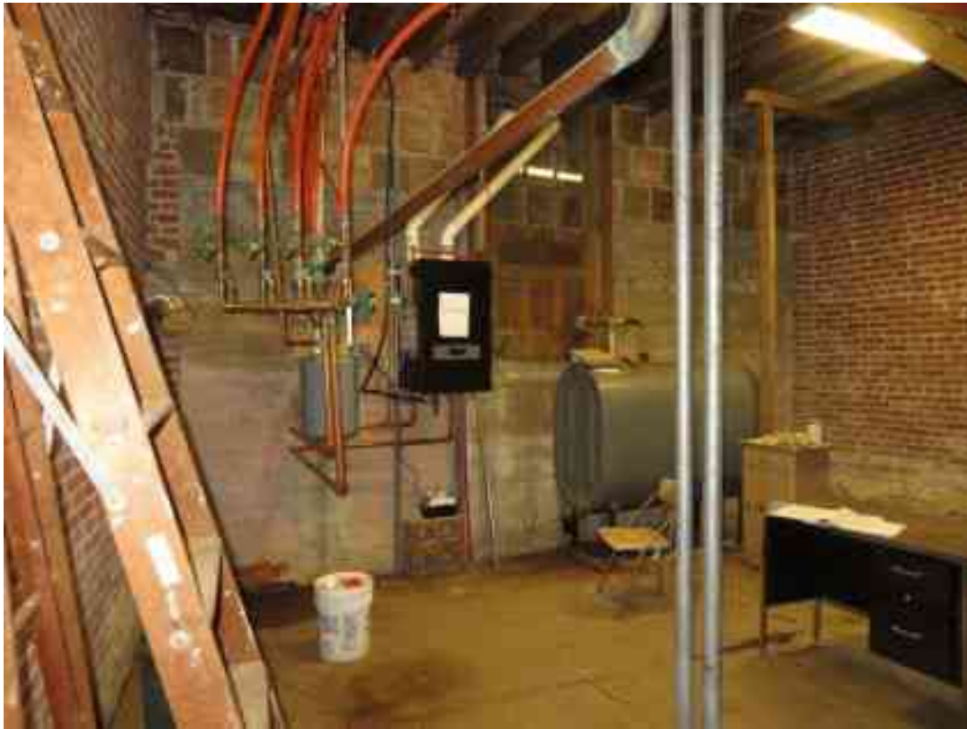
Photo 29: Looking northwesterly in Mechanical Room, basement level. Note concrete foundation and clay tile back-up at exterior walls, and brick interior walls.
