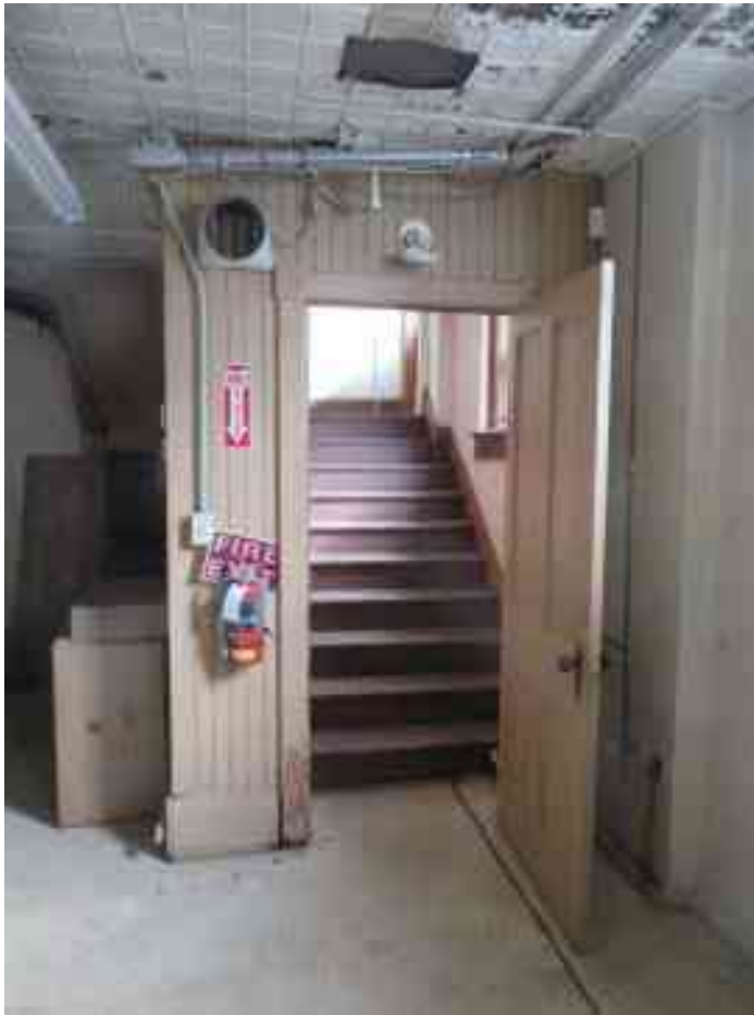
Photo 33: (left) Looking east to enclosed historic stair from basement level.
