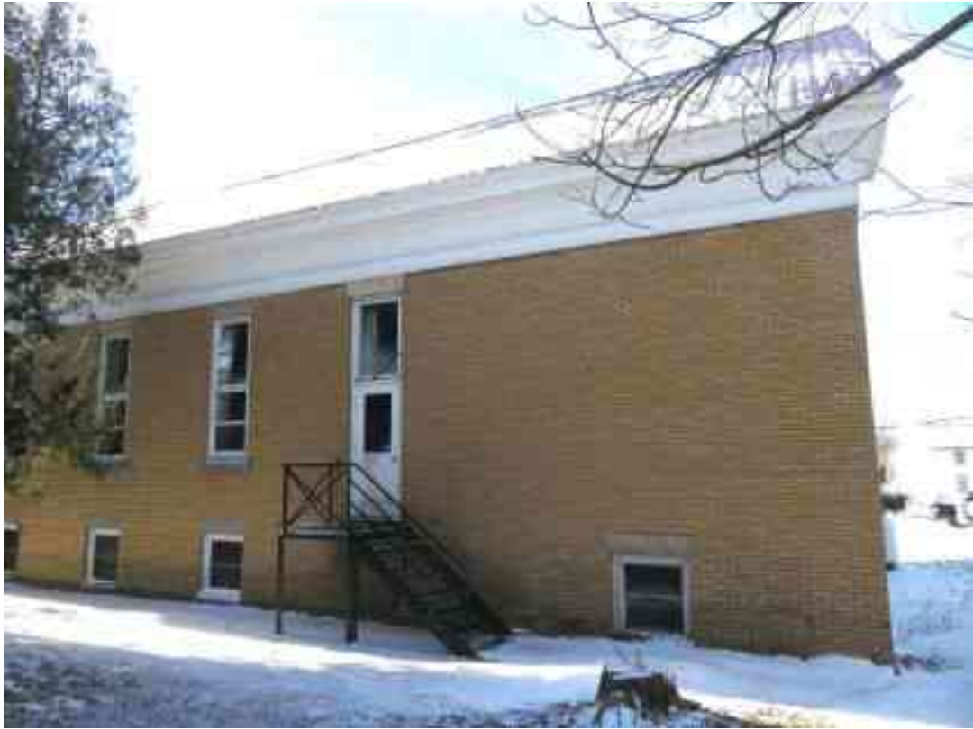
Photo 07: Looking southeast to north face of building. Note metal steps and exit from stage left at theater floor level.
