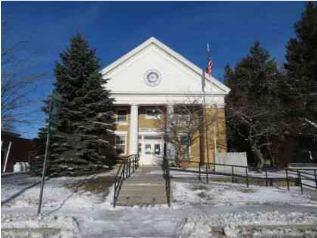
Photo 03: Front (East) elevation. Note concrete walk with ramp for accessibility and veteran's memorial.
