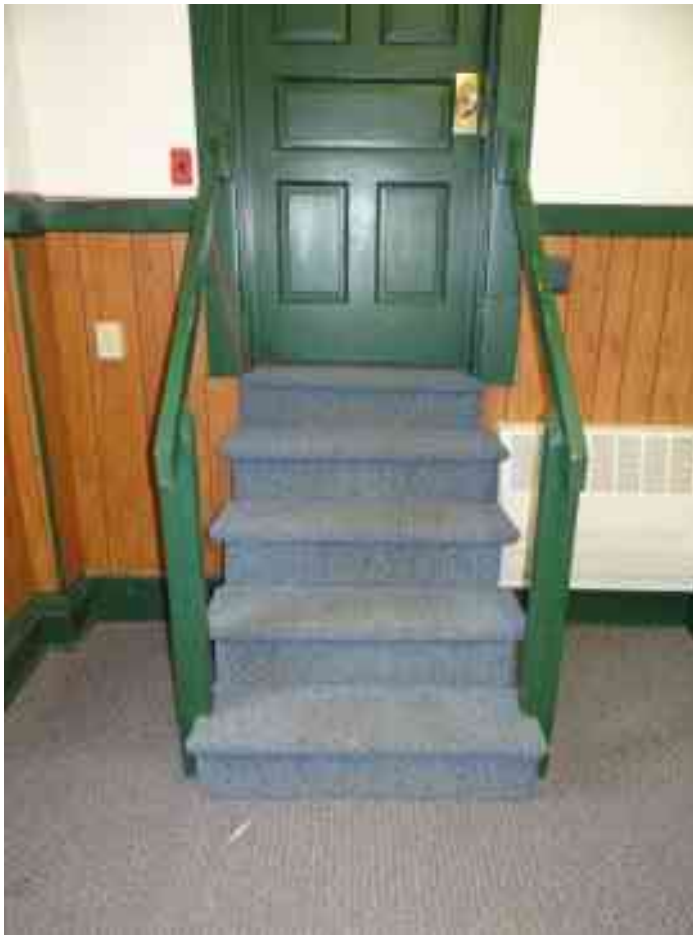
Photo 22: (left) Detail of steps up to former stage from South Room.
