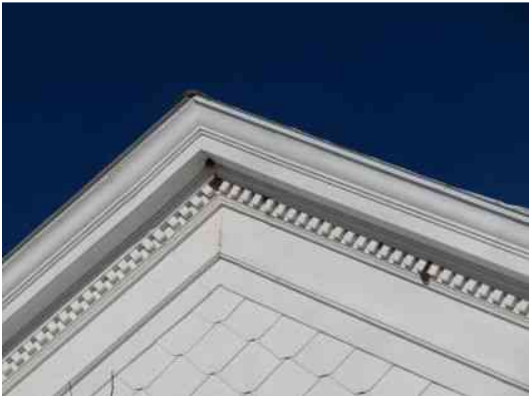
Photo 04: Detail at peak of front gable. Note sheet metal trim with decorative diamond shingles.
