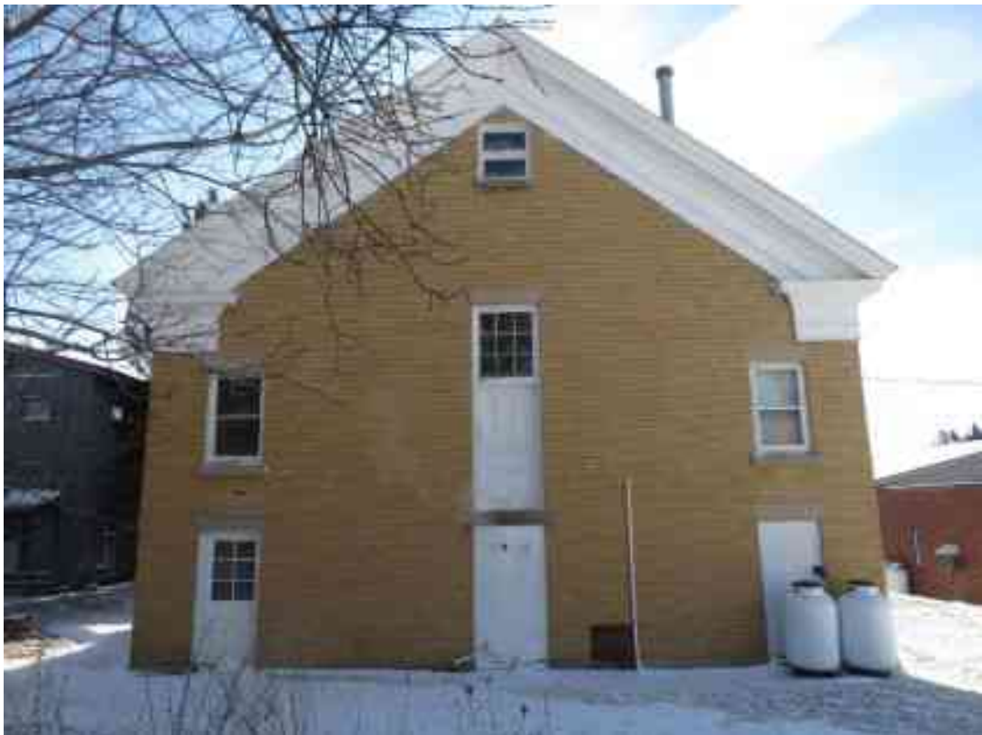
Photo 08: Rear (west) elevation. The “upper” door is located at stage level and the lower doors access stairs down to the basement level.
