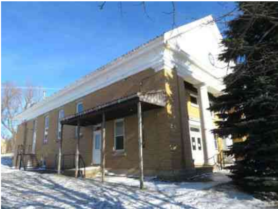
Photo 10: Looking northwesterly to south face of building. Note light framed protective canopy.
