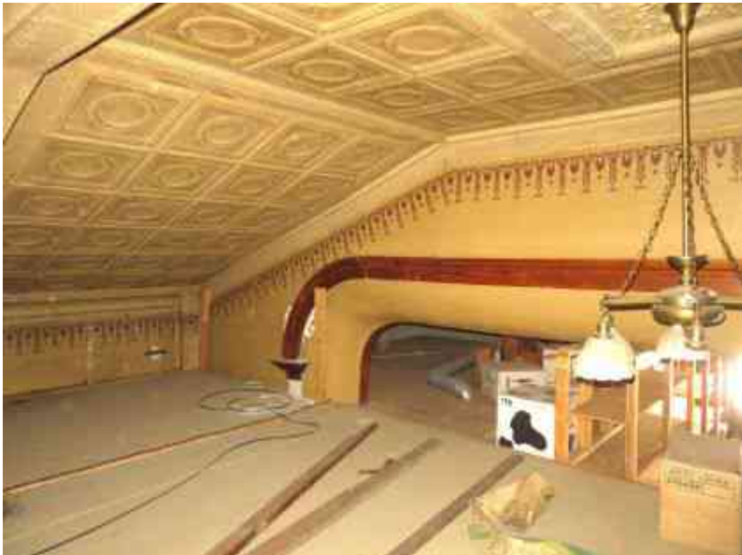
Photo 25: (below) Looking southwest in space above level added within original theater. Note historic features and finishes.
