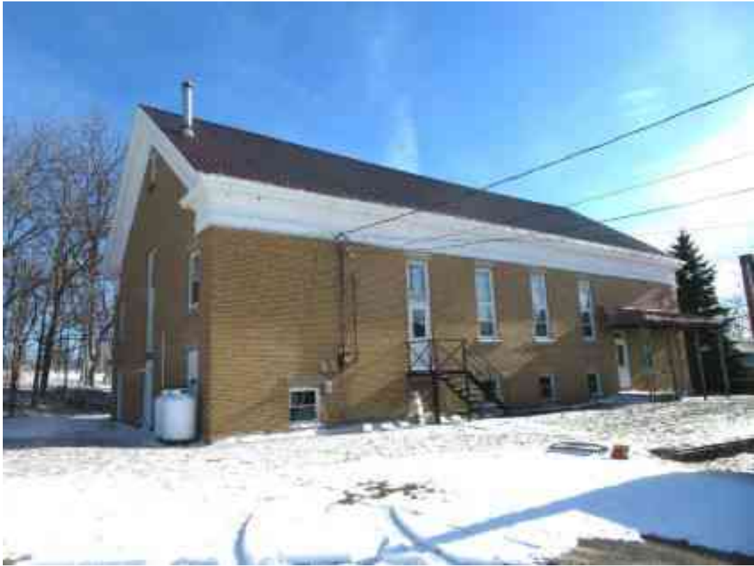
Photo 09: Looking northeasterly to south face of the building. Note exit and metal steps at stage right as well as southeast stair egress beyond.
