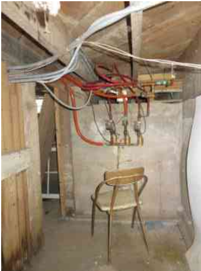
Photo 29: Looking northwesterly in Mechanical Room, basement level. Note concrete foundation and clay tile back-up at exterior walls, and brick interior walls.
