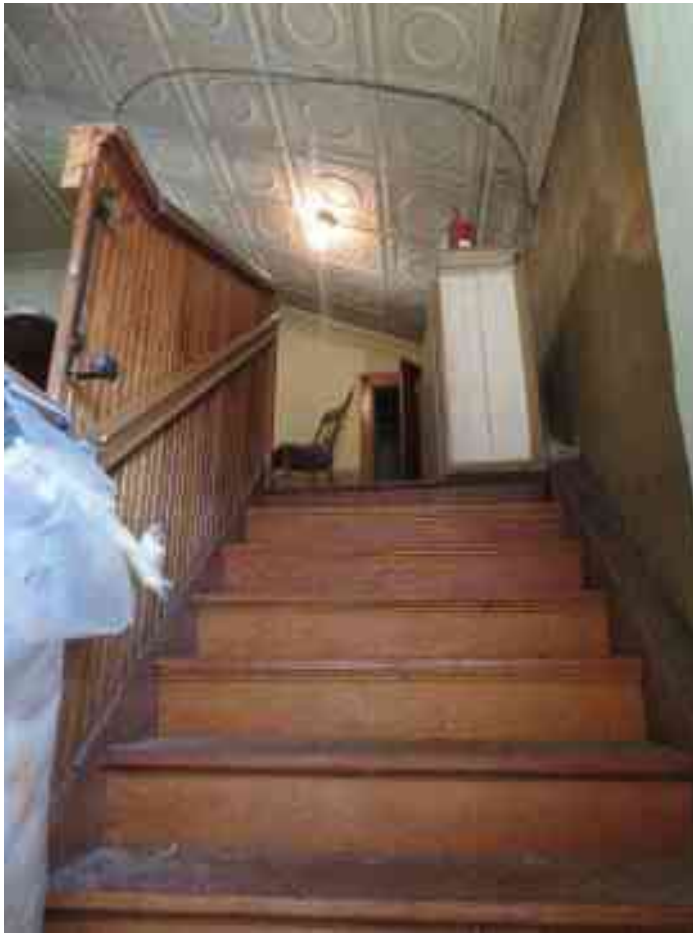
Photo 24: (left) Looking up historic stairs from main level to balcony space.
